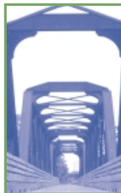
Trestle bridge in Warwick
