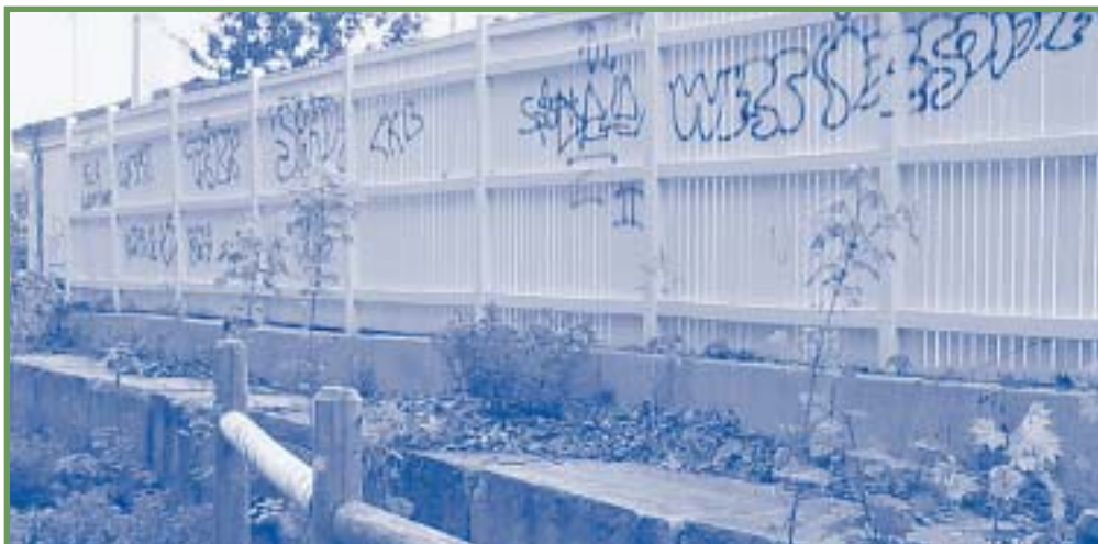
Vandals have been busy on the Cranston Bike Path.
