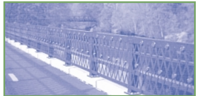
The Albion Mills Bridge offers a nice river view.
